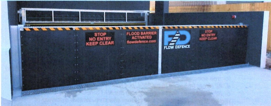
Figure 2 - Typical Flow Defence Hidden Flood Barrier (activated)
